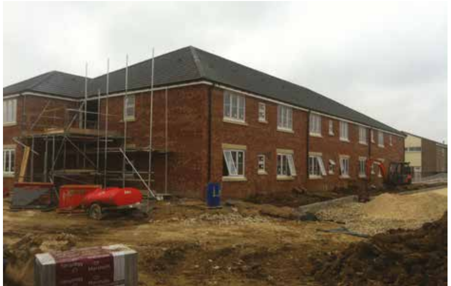
Construction of supported living apartments in Grimsby
